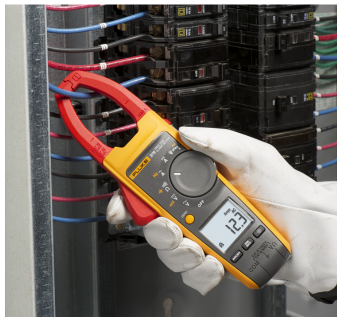
Measuring current with a clamp meter.
