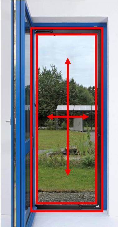
Once the four external braces have been assembled, adjust the frame to loosely fit the dimensions of the door frame (leave about a finger's width on all sides).
